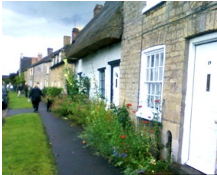
Helpston Cottages. Photograph by Valerie Pedlar.
